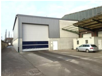
Bielefeld transfer station
